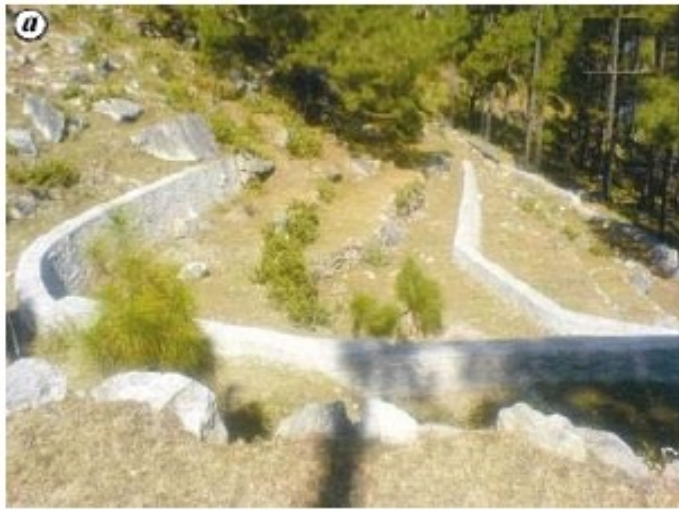
(a) Subsurface dykes; (b), New spring that appeared subsequently. Isotope techniques to identify recharge areas of springs for rainwater harvesting in the mountainous region of Gaucher area, Chamoli District, Uttarakhand.
